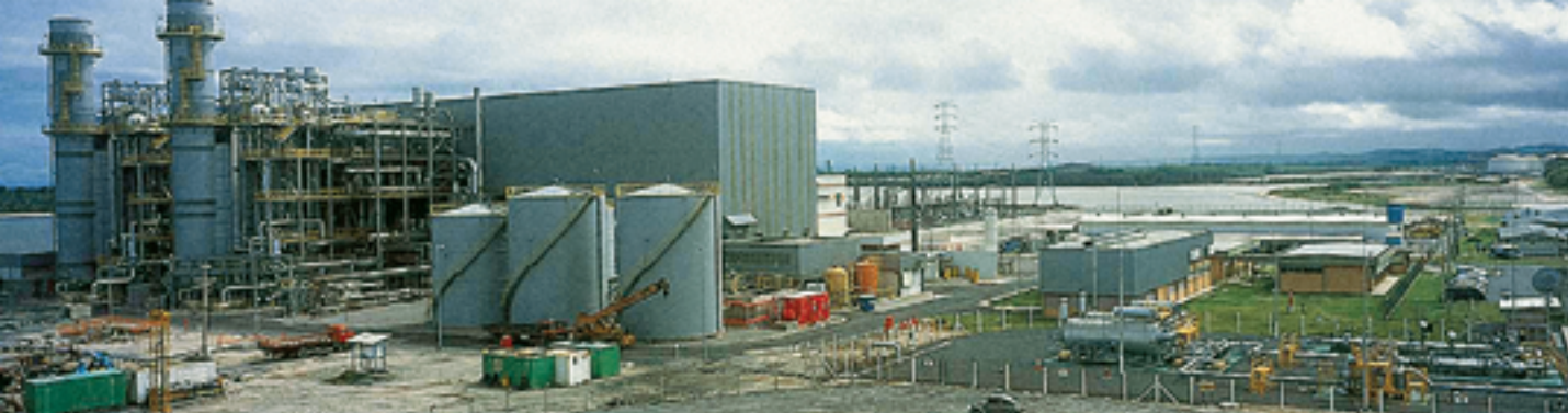
UHE Termopernambuco (PE).
